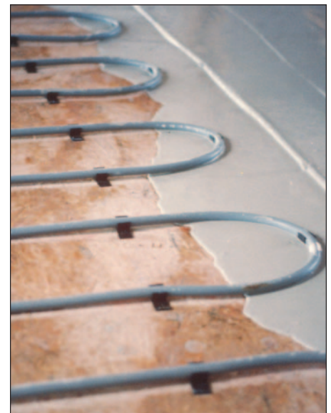
5/8" Tubing installed on top of plywood floor.
